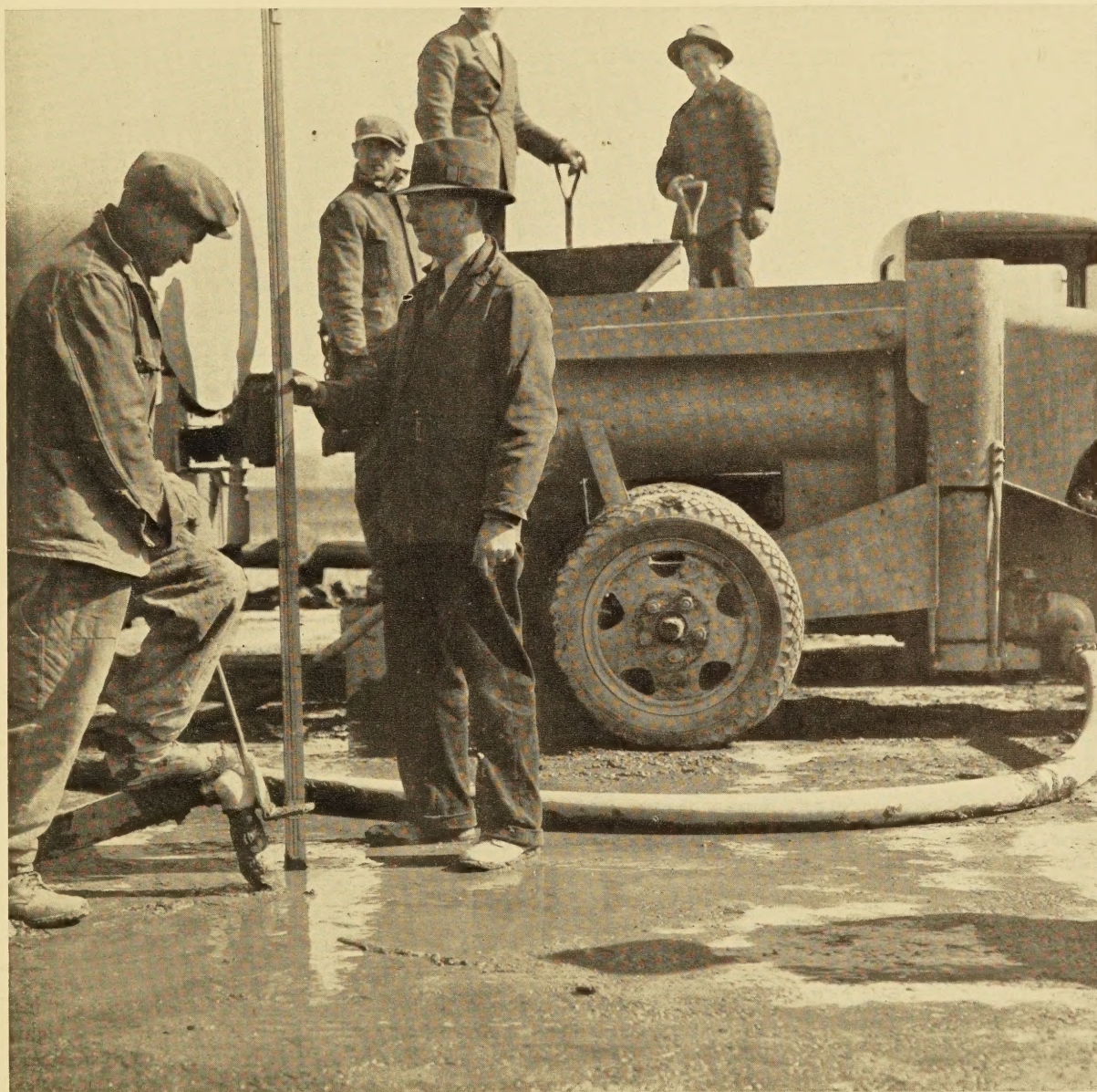
RAISING PAVEMENT BY MUD JACKING
